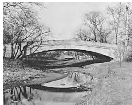
Pleasant Run bridges, Garfield Park
